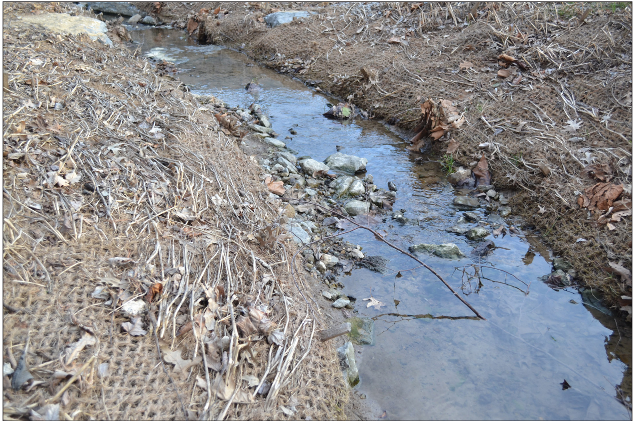
Figure 11. Erosion control blanket made of natural fibers.
